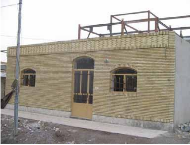
Photo 2: EP house under reconstruction in Bam
