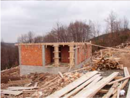
Photo 1: Kosjeric building under construction municipality
