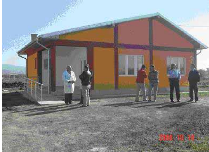
Photo 1: Rehabilitated Health Centre – Autumn 2006
