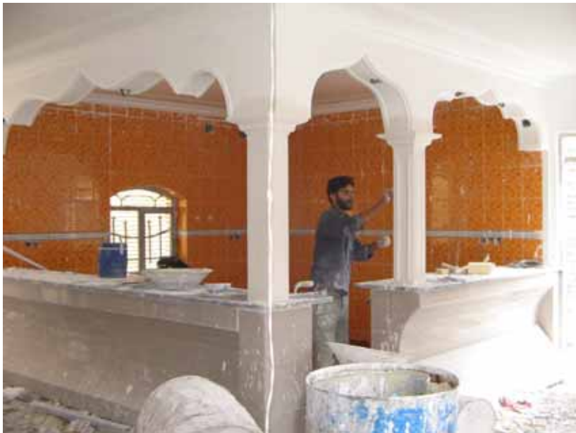
Photo 1: EP house under reconstruction in Bam
