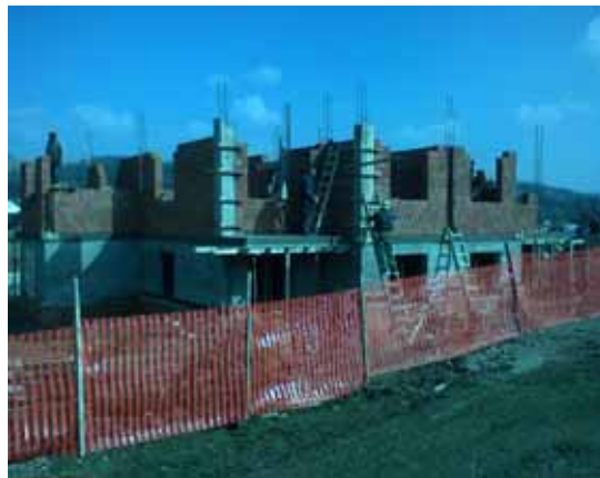
Photo 3: Construction works at Svrlijig apartment block
